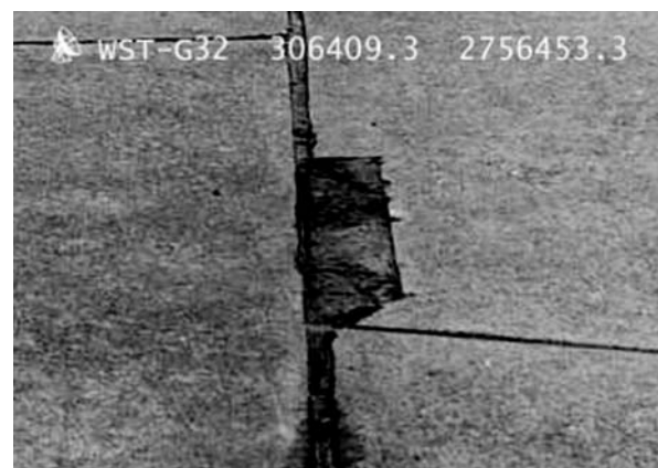
Fig. 7. Automatically acquired pavement images.
