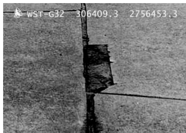
Fig. 7. Automatically acquired pavement images.
