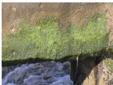
Fig. 1. Growth of marine seaweed on structural components.
