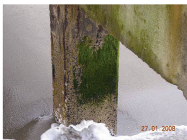
Fig. 3. Growth of marine seaweed on structural components.
