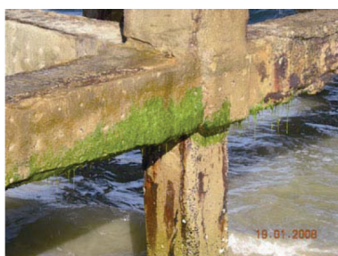
Fig. 2. Growth of marine seaweed on structural components.
