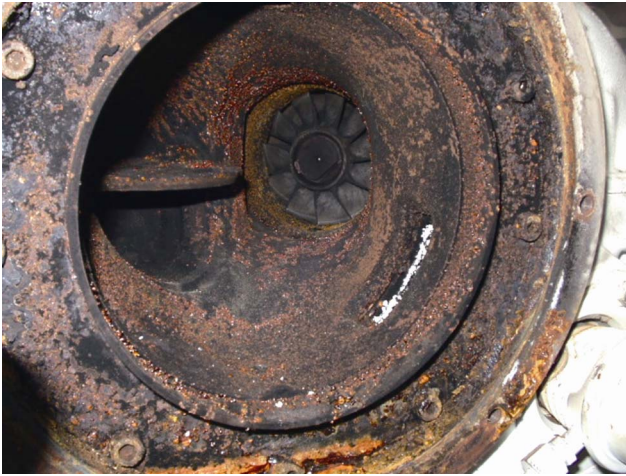
Fig. 5. Rust and corrosion signs at the exhaust turbocharger outlet.
