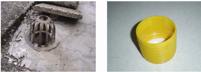
Fig. 4. Rooftop drain outlet and capping device.
