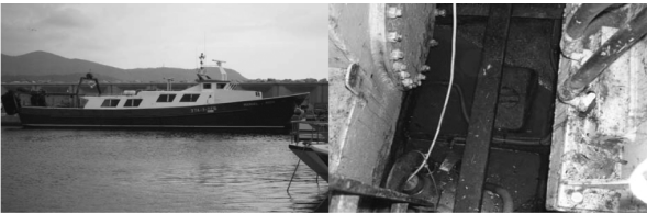
Fig. 20. Gradual corrosion of the steel hull.
