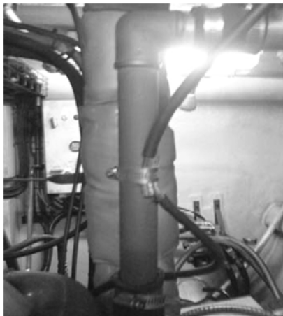
Fig. 26. Corrosion failure to protect main engine and pipes.
