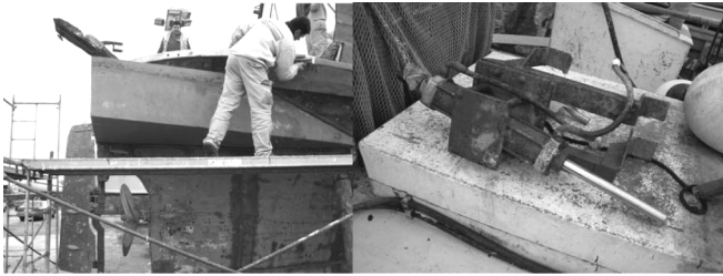
Fig. 13. Corrosion in steel rudders and servo drive components.
