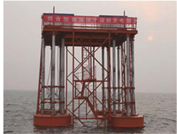
Fig. 7. The 10 kW combined oscillating buoys WEC developed by OUC.
