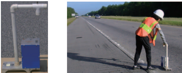
(a) The Georgia fault meter (b) Manually measure faulting on the roadway
