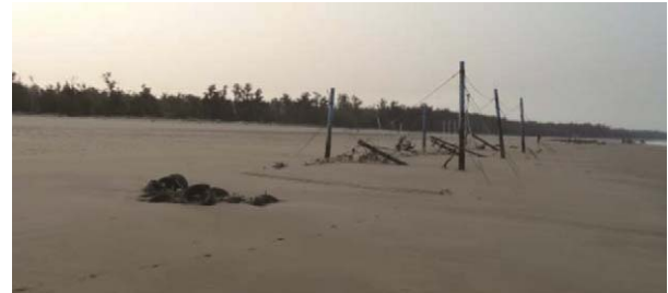
Fig. 11. Beach appearance on 2011/10/04, approximately 2 yrs after the set-up of device No. 1. Rich sedimentation can be seen around the breakwater.
