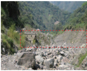
Fig. 8-1. Sabo dam NO. 1.
