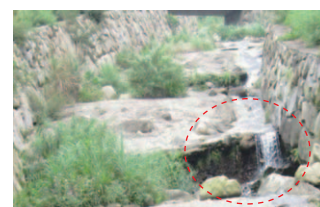
Fig. 7-2. Groundsill work NO. 2.
