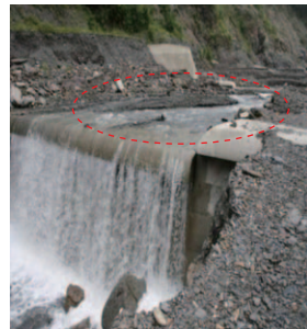
Fig. 8-2. Sabo dam NO. 2.
