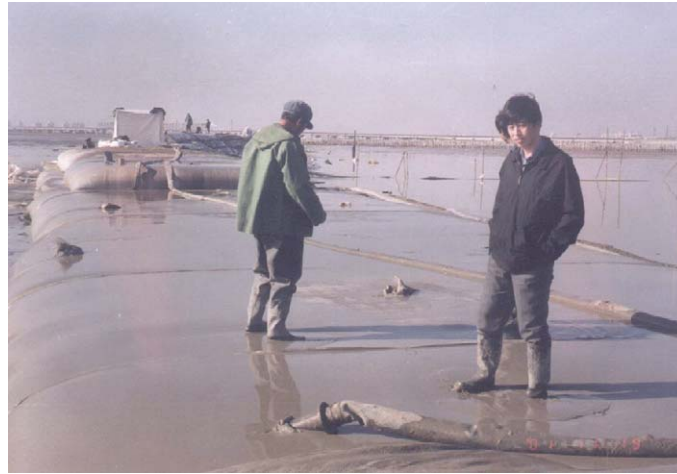
Fig. 1. Geosynthetic bag in filling.
