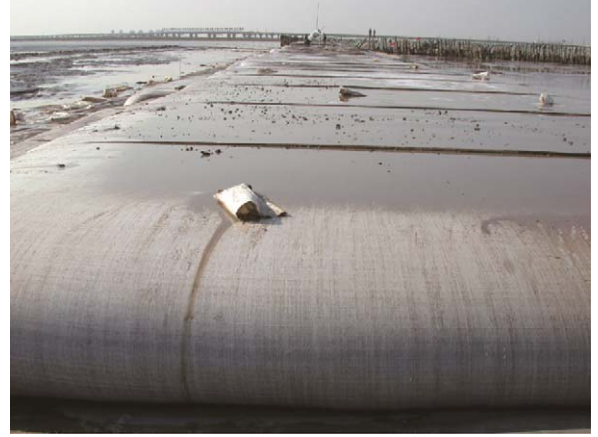
Fig.16. Shape of a partially inflated geotube.
