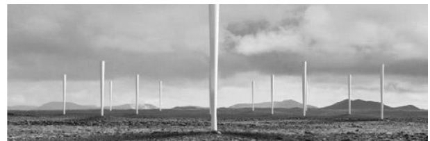
Fig. 1. The vortex wind generator developed by Vortex Bladeless (2015).
