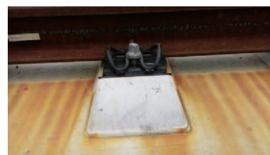
(b) rail fastening device
