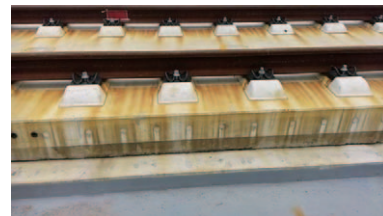
(a) non-ballasted slab track
