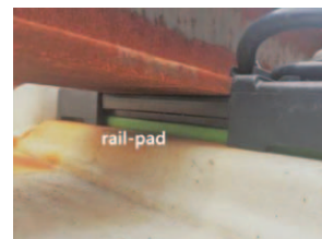
(c) rail-pad with rubber material
