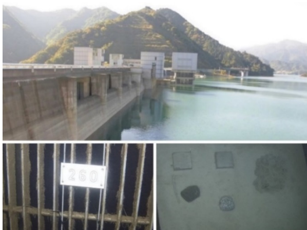
Fig. 10. Top: Target dam, lower left: Penstock intake, lower right: image at a depth of about 100m – to confirm camera resolution
